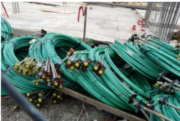
Post-tensioning Cables
