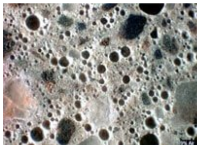
Air-Entrained Concrete, Photo credit: Portland Cement Association (PCA)
