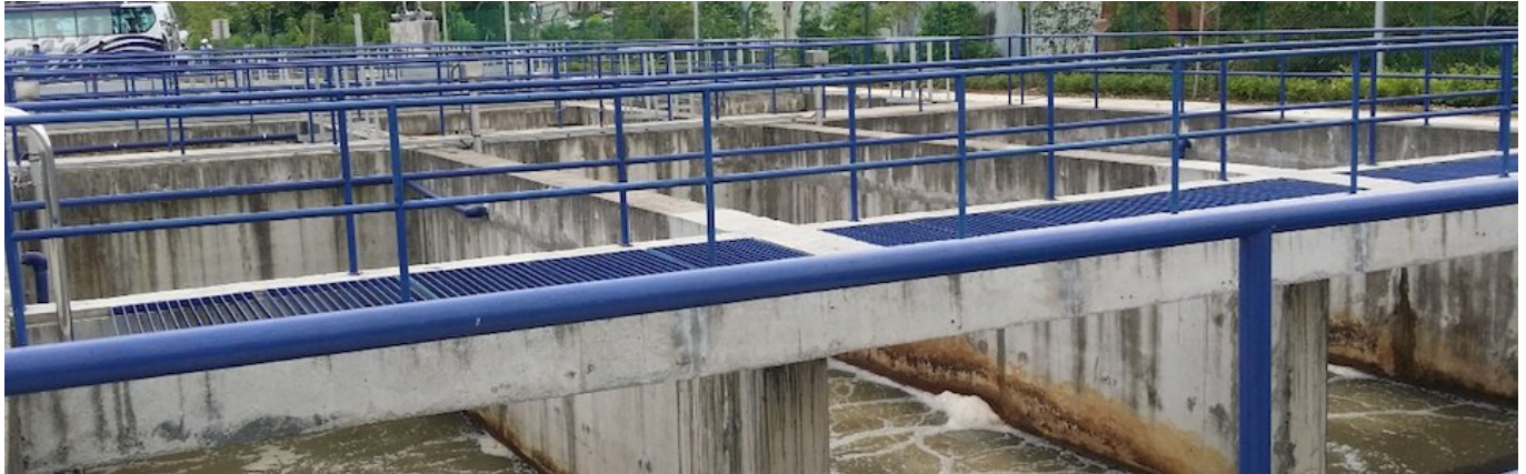
River Water Treatment Plant in UKAY Perdana, Ampang
