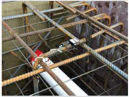
SmartRock<sup>™</sup> sensors installed on rebar
