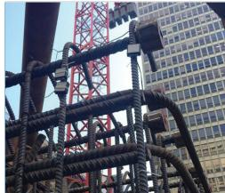
SmartRock<sup>™</sup> sensors attached to rebar
