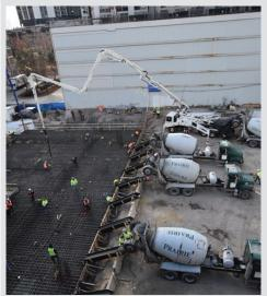
Continuous mass concrete pour over SmartRock™ wireless sesors installed on rebar
