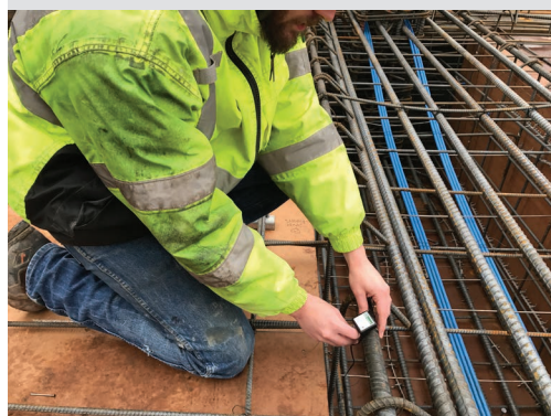
Construction worker installing SmartRock Plus sensor on rebar
