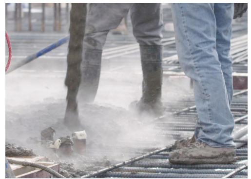
SmartRock2 sensors are fully embedded in concrete during construction
