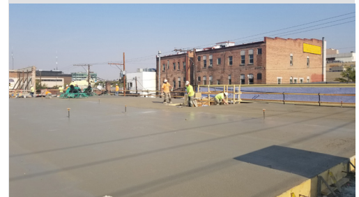
Construction workers collecting concrete temperature strength data after pouring.
