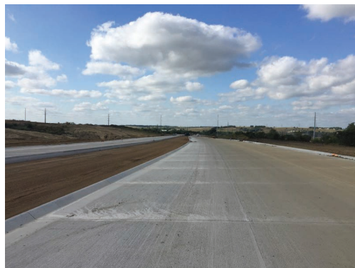
Completed Concrete Highway
