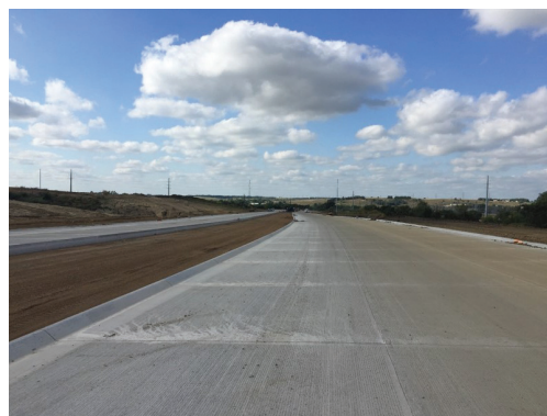
Completed Concrete Highway
