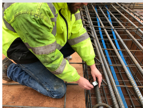
Construction worker installing Smart Concrete sensor on rebar
