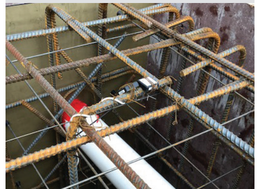
SmartRock2™ sensors installed on rebar
