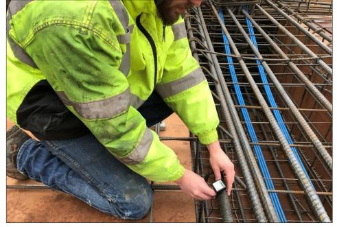
Giatec Scientific's 2-by-2-inch sensors can be placed in concrete to send information about its strength and temperature in real time. A smartphone app can read the data. Photo courtesy of Stoneway Concrete
