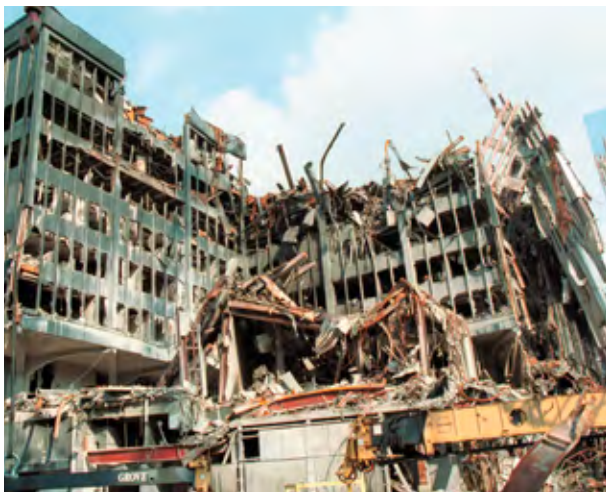
An example of concrete infrastructure in America not being repaired or sustained.
