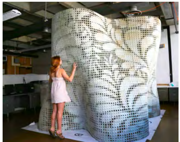
'Bloom' the 3D printed structure created by the University of California Berkeley.
