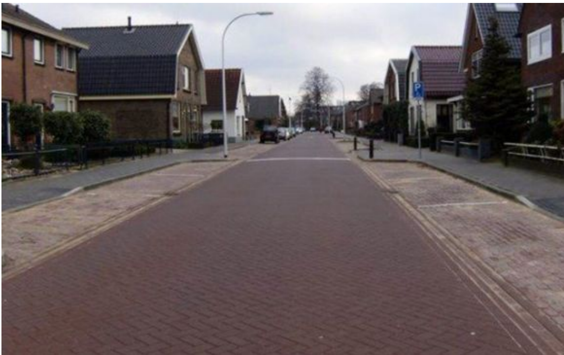
A street in the Netherlands paved with smog-eating concrete
