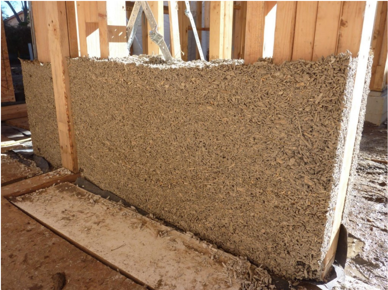
An example of a wall made with hemp concrete
